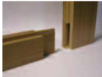
Mortice and tenon joint
